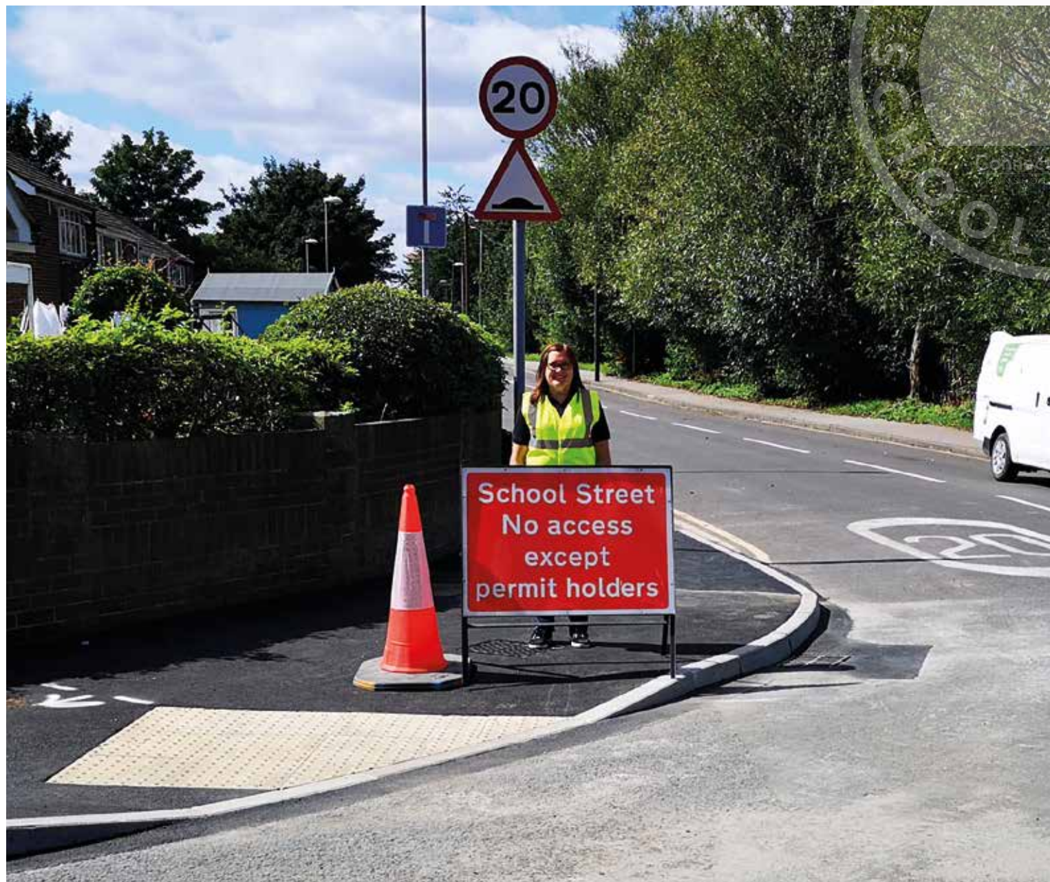
Figure 3: Temporary 'No Access' sign as illustrated in School Information Pack
